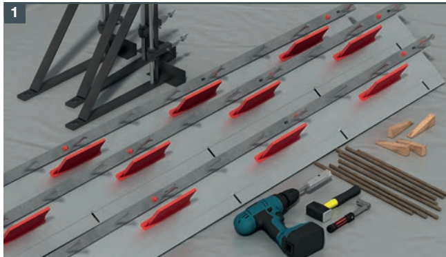
1 Set up the site. Laser dumpy level set up, finished floor level datum taken, membrane laid, hand tools available
