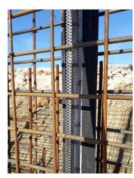
The use of the CEMFLEX VB metal sheet is covered by the ETA  $n^{\circ}16$  /0601 (European Technical Assessment) and the DTA 3.3/19-1006\_V1 (CSTB) which guarantees the waterproofing of the concrete up to a pressure of 2 bars, i.e 20m of water pressure.
