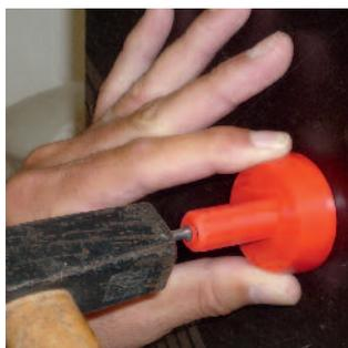
Easily nail clamping flange to the wooden shuttering
