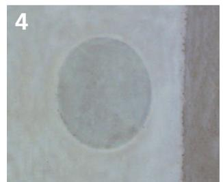
*Glue in fine-grained cone, perfect result for high exposed concrete!*
