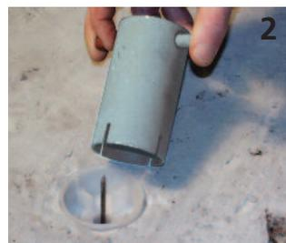
*Removing of clamping flange with removing tool*
