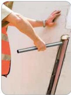
Deploy the standby steel reinforcements. It is important not to create a bayonet effect. To do this, use the deploying tool and jog the tool forward as close as possible to the curvature.
