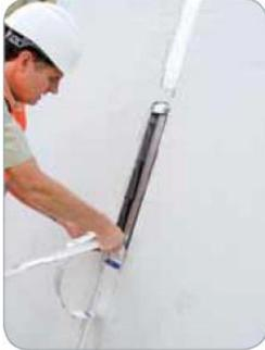
After stripping, remove the cover and plugs from the Stabox.
