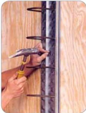
Fasten the Stabox to the formwork and/or the reinforcement if applicable. When using a type S Stabox (single strand) add ligatures or in specific cases include spacers for proper anchoring.
