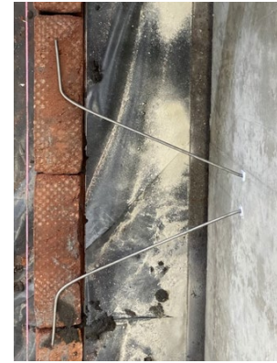
Photo 7: Ancrage sismique
