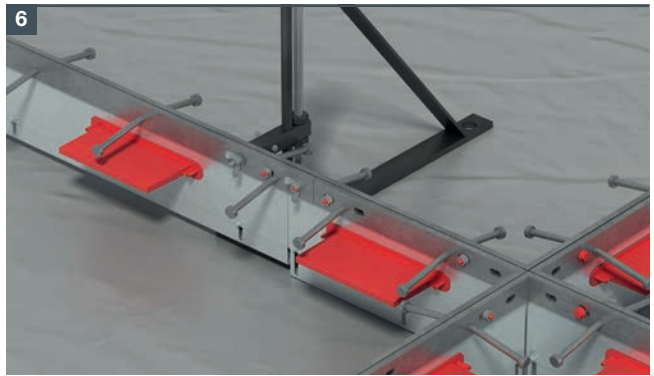
6 Continue to fit the ArmourJoints. Ensure the lapped joints are butted end to end tightly. Fit the plastic bolt and wing nut at the lapped joint.
