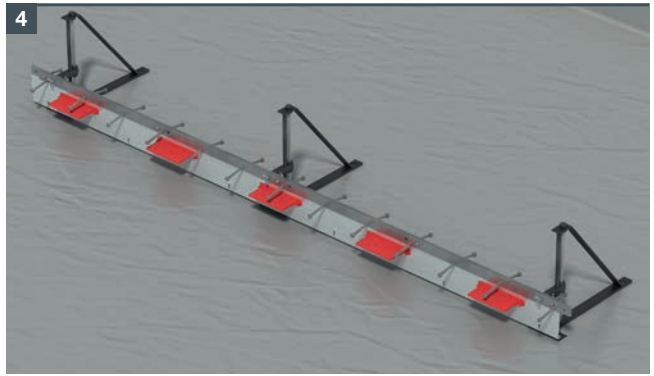
4 Fit ArmourJacks to the ArmourJoint top strips.
