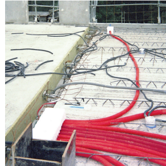
2 Phase 1 concreting and Phase 2 Titan dowel positioning. The springs are positioned.
