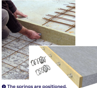
2 The springs are positioned.
