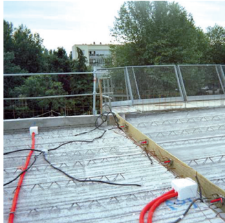
1 Phase 1 Titan dowel positioning.
