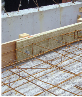
1 The strips are nailed to the edge formwork.
