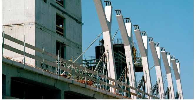
FIXING AND ADJUSTING PRECAST ELEMENTS
